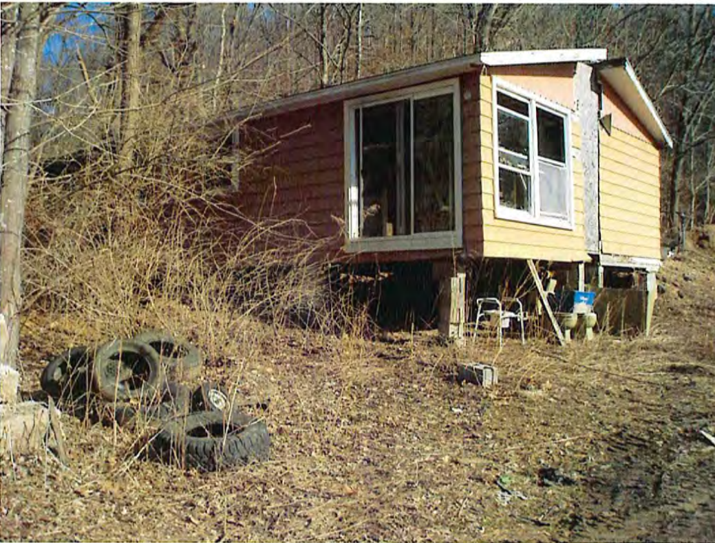
Date: 1/3/2014 Time: 1:00 P.M. Direction: southeast Photo by: S. Williams Exposure #: 014 Comments: two toilets, portable toilet, tires, and two halves of a house placed together and positioned on concrete blocks
