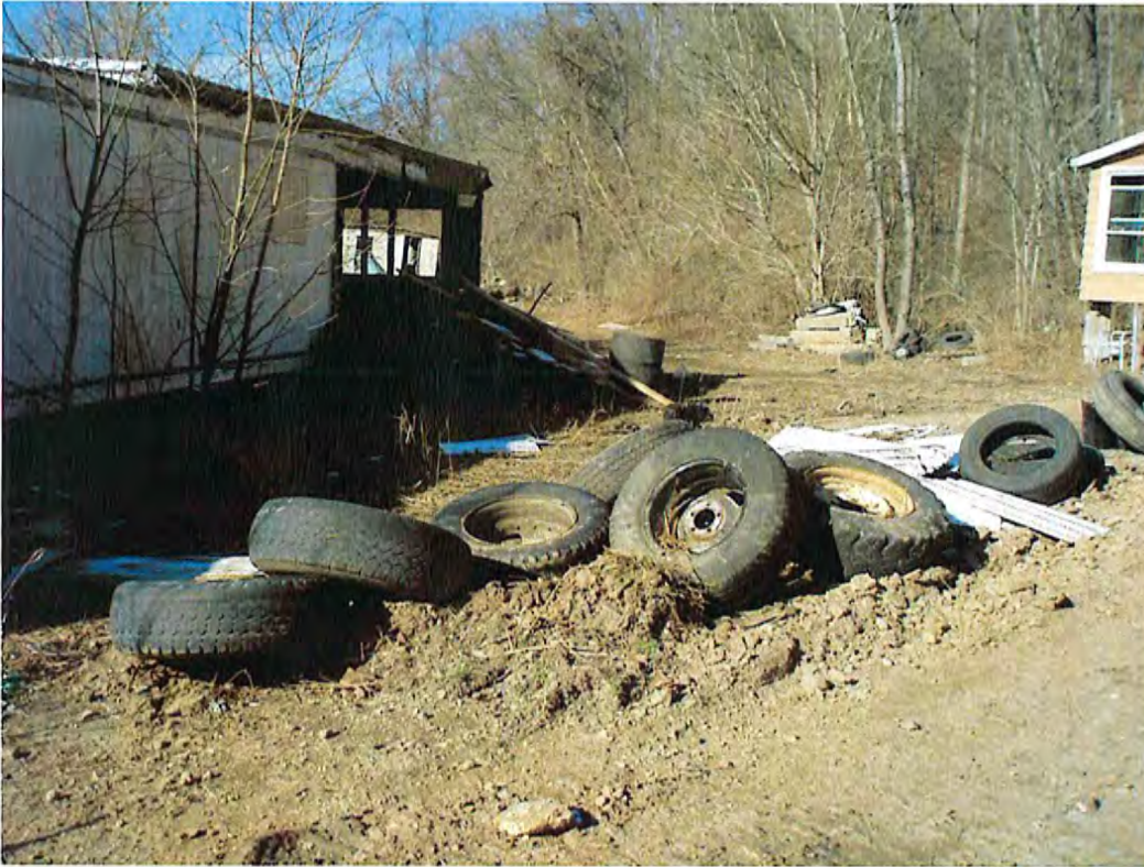
Date: 1/3/2014 Time: 1:11 P.M. Direction: north Photo by: S. Williams Exposure #: 021 Comments: tires and demolition debris
